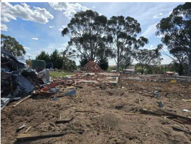
Photograph 3 – Footprint of demolished house (looking west) with slab centre picture and piles of C&D waste remaining on-site (bricks and steel in background and corrugated metal sheeting in foreground left).
