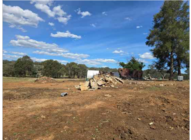
Photograph 2 – Footprint of demolished Shed 3 looking south with C&D waste (concrete) and former UST in centre picture.
