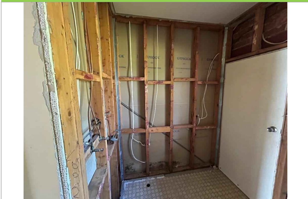
Photograph 5: Photograph following removal of ground floor bathroom wall sheet
