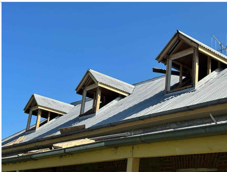
Photograph 10: Photograph following removal of Infill panels to attic windows
