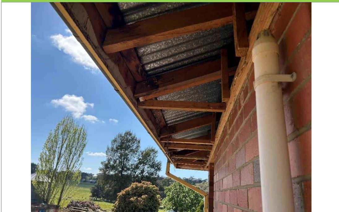
Photograph 7: Photograph following removal of external eave lining
