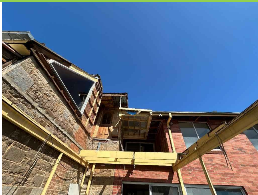
Photograph 9: Photograph following removal of veranda floor sheet
