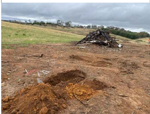
Photograph 15 – Ground conditions around TP13, noting C&D waste (wood and steel) pile to the east
