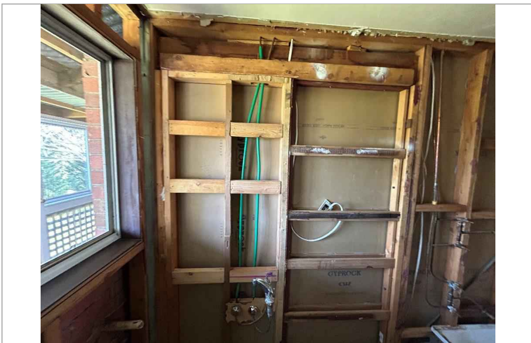
Photograph 6: Photograph following removal of first floor bathroom wall sheet
