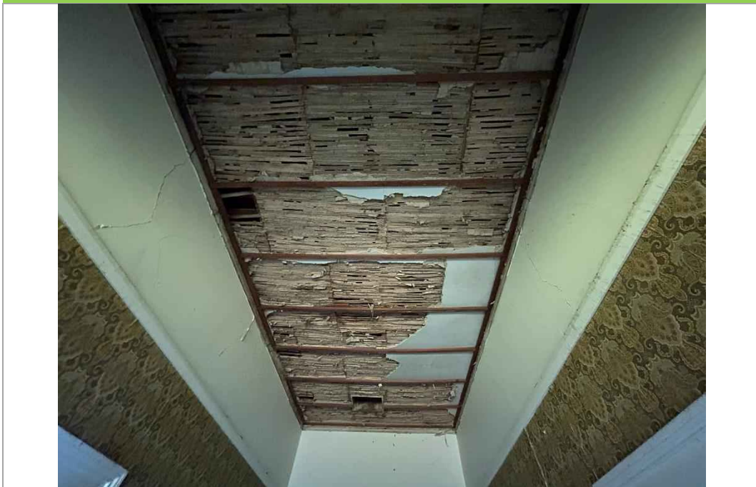
Photograph 1: Photograph following removal of ceiling sheet to front entry
