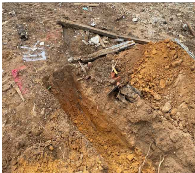
Photograph 16 – Ground conditions at TP17 with natural soils encountered at surface, noting remnant demolition waste at surface.
