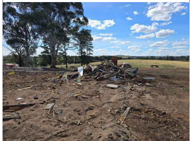
Photograph 4 – Footprint of demolished Shed 1 looking north with C&D waste (steel and wood) in centre picture.
