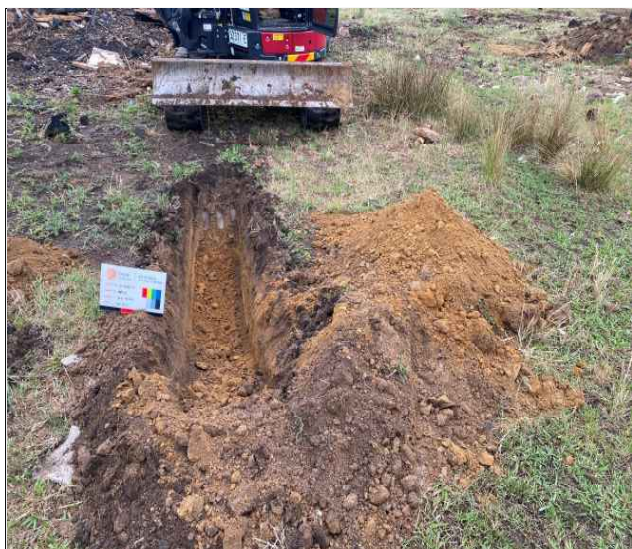
Photograph 13 – TP06 ground conditions, with natural soils encountered approximately 0.3 m BGL with waste piles in background.
