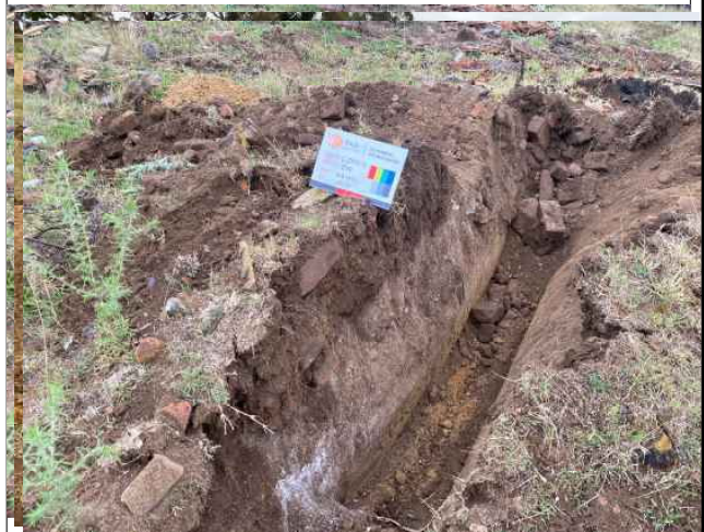
Photograph 6 – C&D waste (brick) extending to approximately 1.0 m BGL in TP07.
