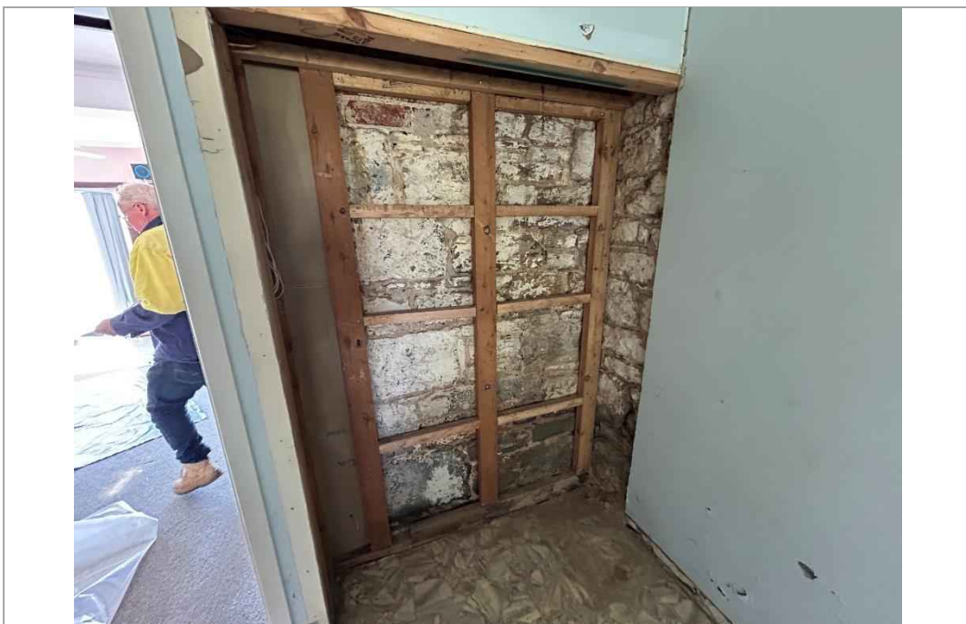
Photograph 4: Photograph following removal of kitchen cupboard lining
