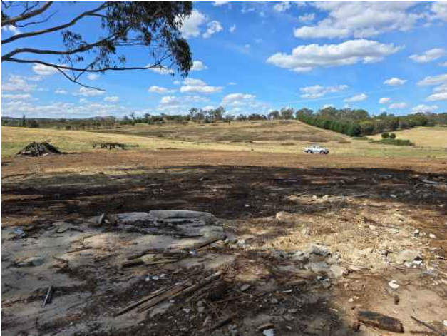
Photograph 1 – Footprint of demolished Shed 3 looking east with remnant slab in foreground.
